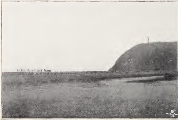
DURBAN BREAKWATER. (SHOWING CHAIN GANG.)
